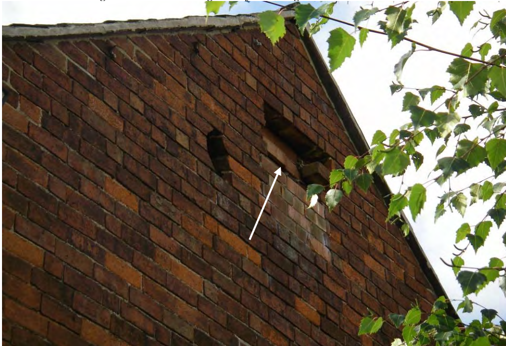
Plate 3.7: Roosting location on north gable of Building 2
